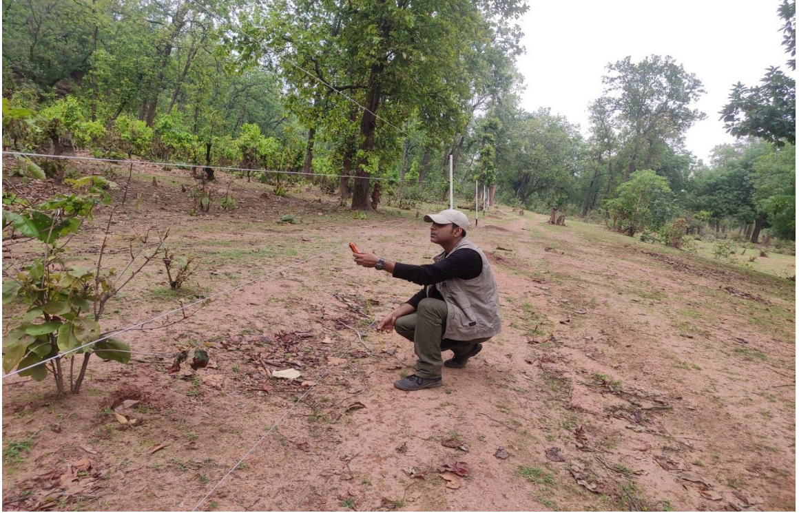
Fencing Voltage Testing
